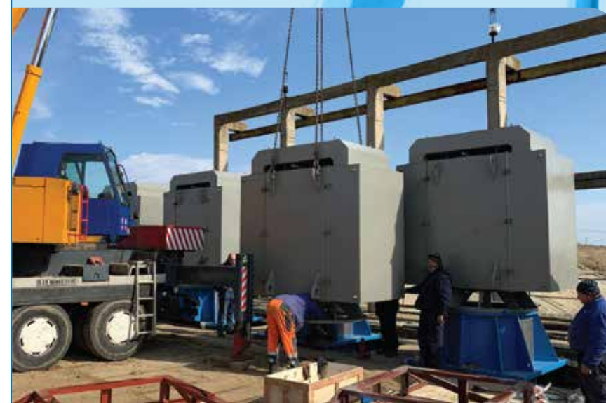
11 Axial Flow Pumps In Ialomita - Calmatui Irrigation Project - Romania 2019 [Over 15.000 M 3 /h]
